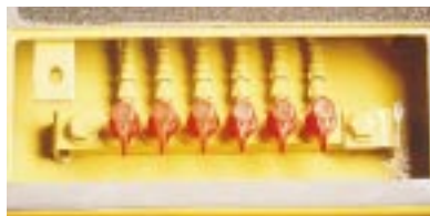
3) Oil Pressure Inspection Ports
